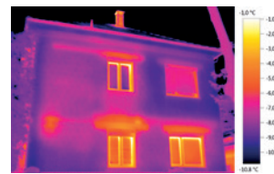
Thermal image with ScaleAssist
